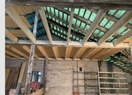
Neue Deckenebene DG/Spitzboden
